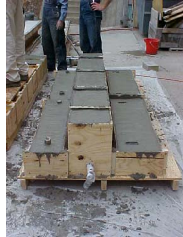
(b) Beams casting
