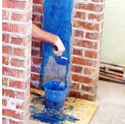
Fig. 3.7. Application of the second coat of saturant
