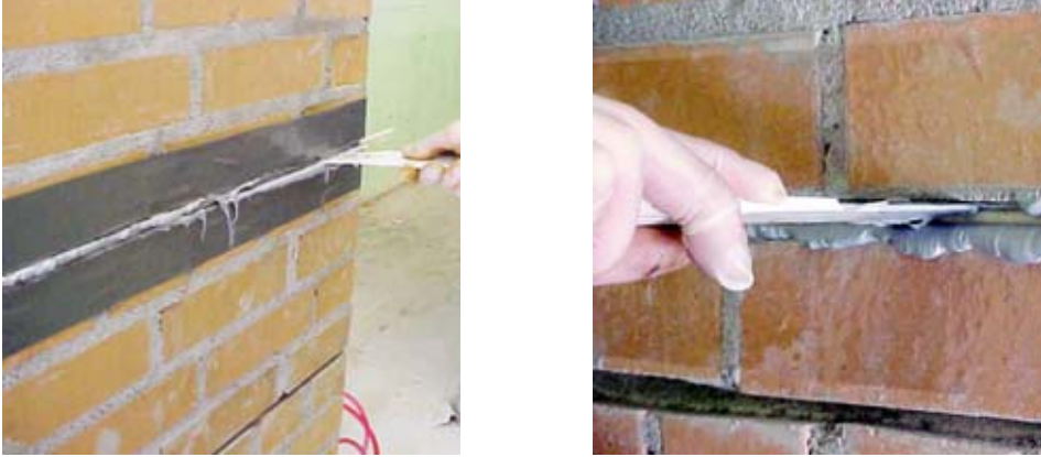
Fig. 3.12. Drawn of the bar into the epoxy-based paste
