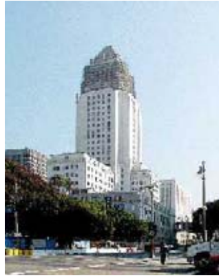
Fig. 1.2. Los Angeles City Hall Building (California)
