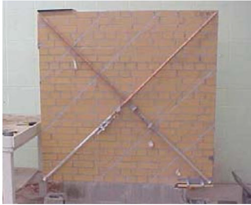
Fig. 6.21. Wall CLW6 after failure (front)
