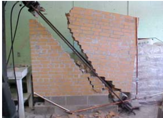
Fig. 6.11. Wall CLW1 after failure (front)
