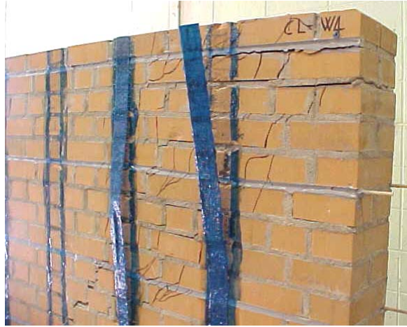
Fig.B.4 - 3. Delamination of GFRP laminates
