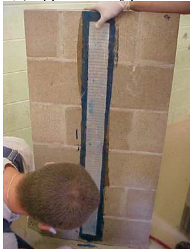
(c) Application of GFRP sheet
