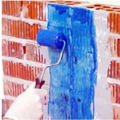
Fig. 3.4. Application of the first coat of saturant
