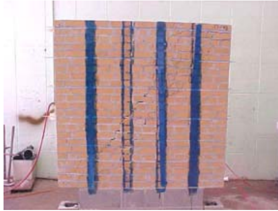
Fig. 6.17. Wall CLW4 after failure (front)
