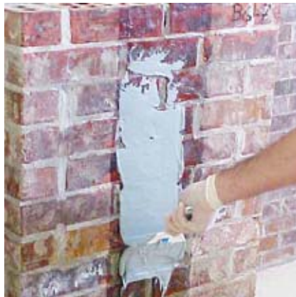
Fig. 3.3. Application of the putty
