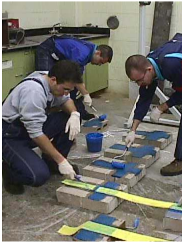
(c) Application of AFRP sheets
