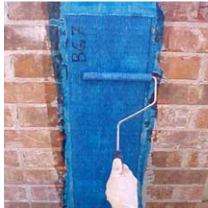
Fig. 3.8. Final removing of the air bubbles
