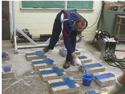
(b) Application first coat of saturant
