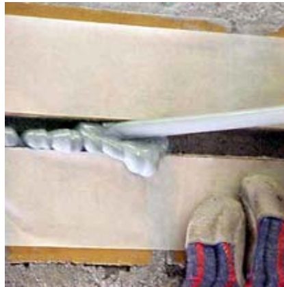
Fig. 3.11. Placing the epoxy-based paste into the slot
