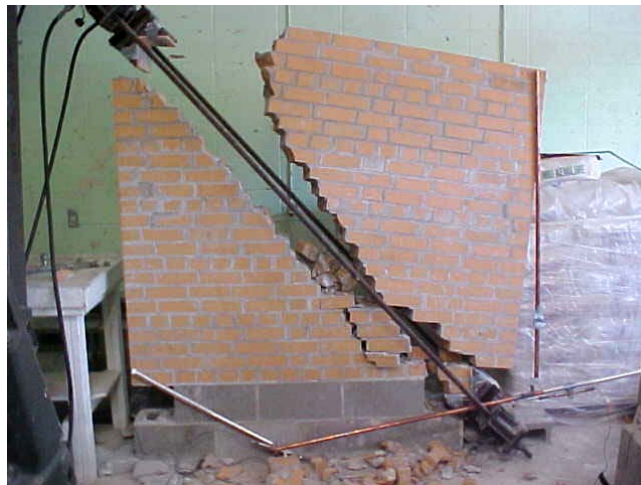
Fig.B.3 - 3. Wall CLW1 after failure (front)
