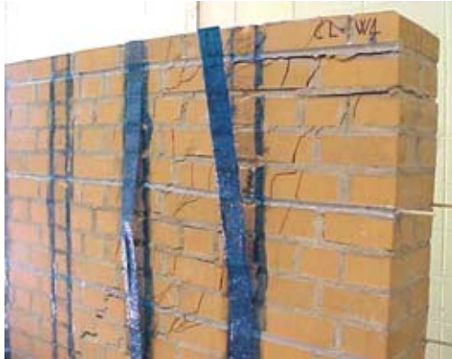
Fig. 6.24. Delamination of GFRP laminates
