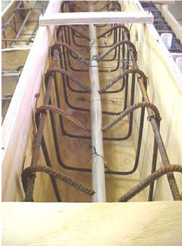
(a) Steel cage and PVC pipe
