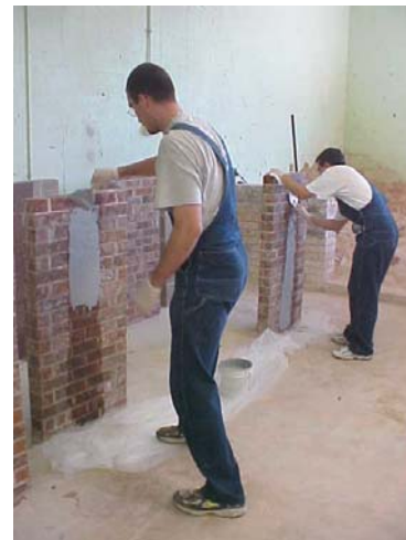
(b) Application of putty
