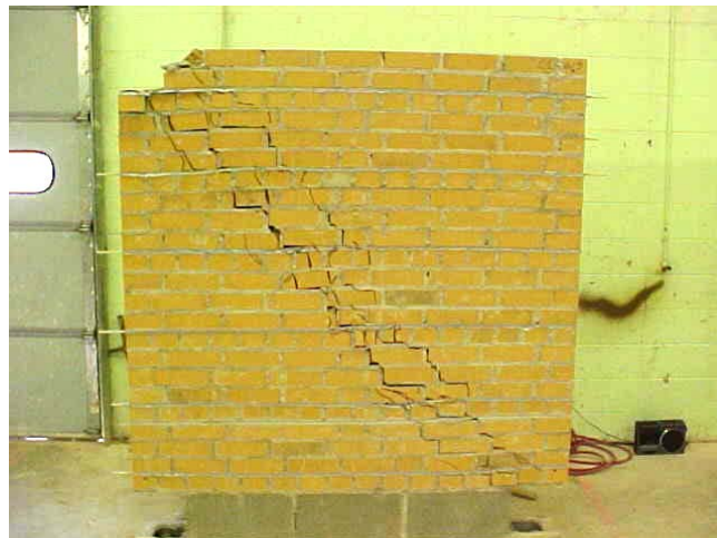
Fig.B.3 - 6. Wall CLW2 after failure (front)
