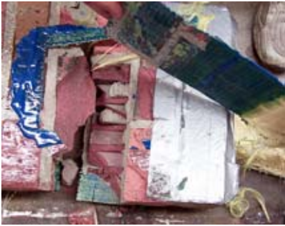
(e) Damage in the masonry bricks
