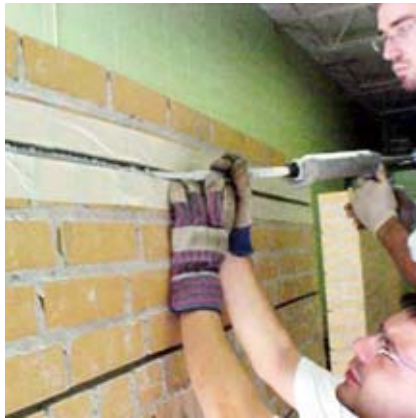
Fig. 3.11. Placing the epoxy-based paste into the slot
