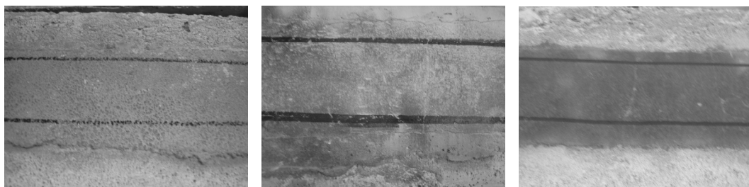
Figure 2. Surface preparation (left to right: Verticoat Supreme, TPM723, & Burke V/O Patch).
